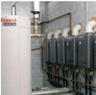
DD6 Internal Flued System
