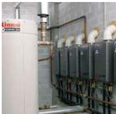
DD6 Internal Flued System
