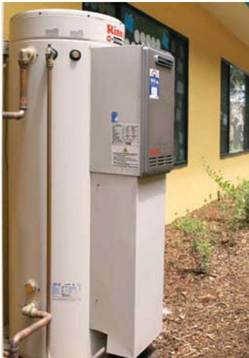
DD1 200 External installed in a narrow sideways
