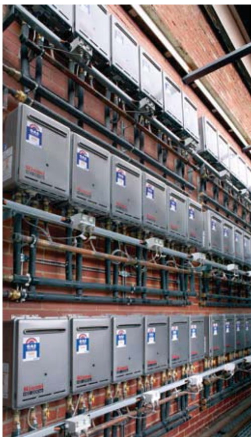
Compact installation of 6 x Manifold Pack 6 External
