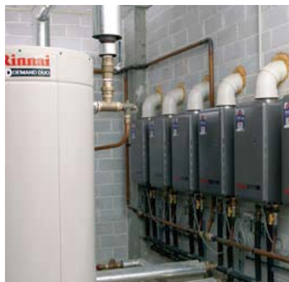
DD6 Internal Flued System
