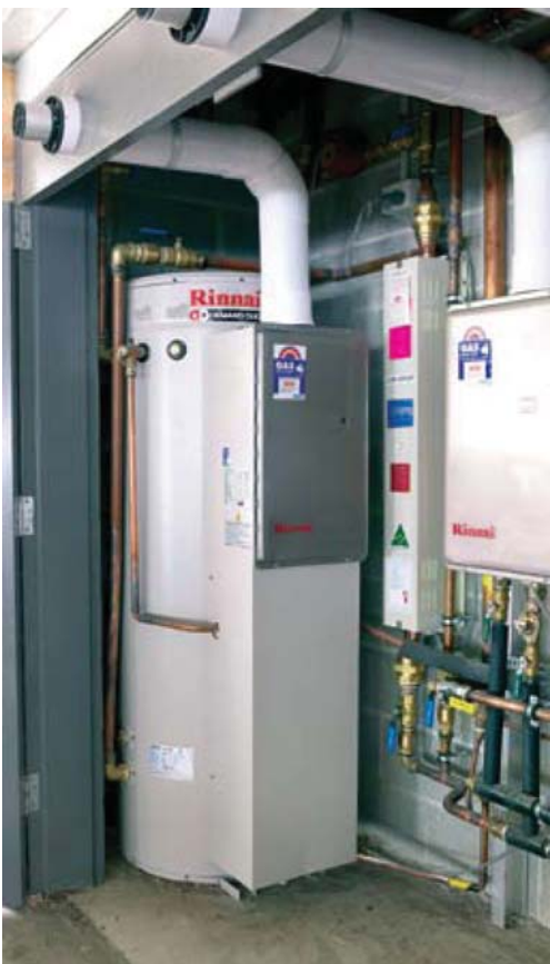
DD1 200 Internal installed in a cupboard
